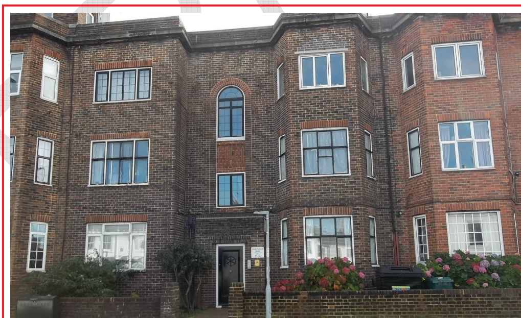
Variety of window styles, opening arrangements, materials and colours harmful to appearance of building
